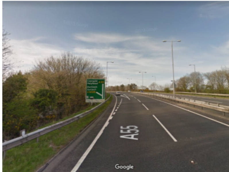
Exit 8 on A55 Expressway - A5025 Benllech
